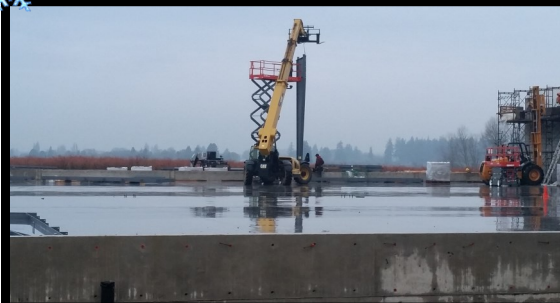
First structural beam going up for the new facility
