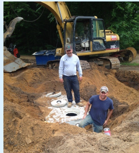
Buddy supervising Scott's work on Krader septic tank installation.
